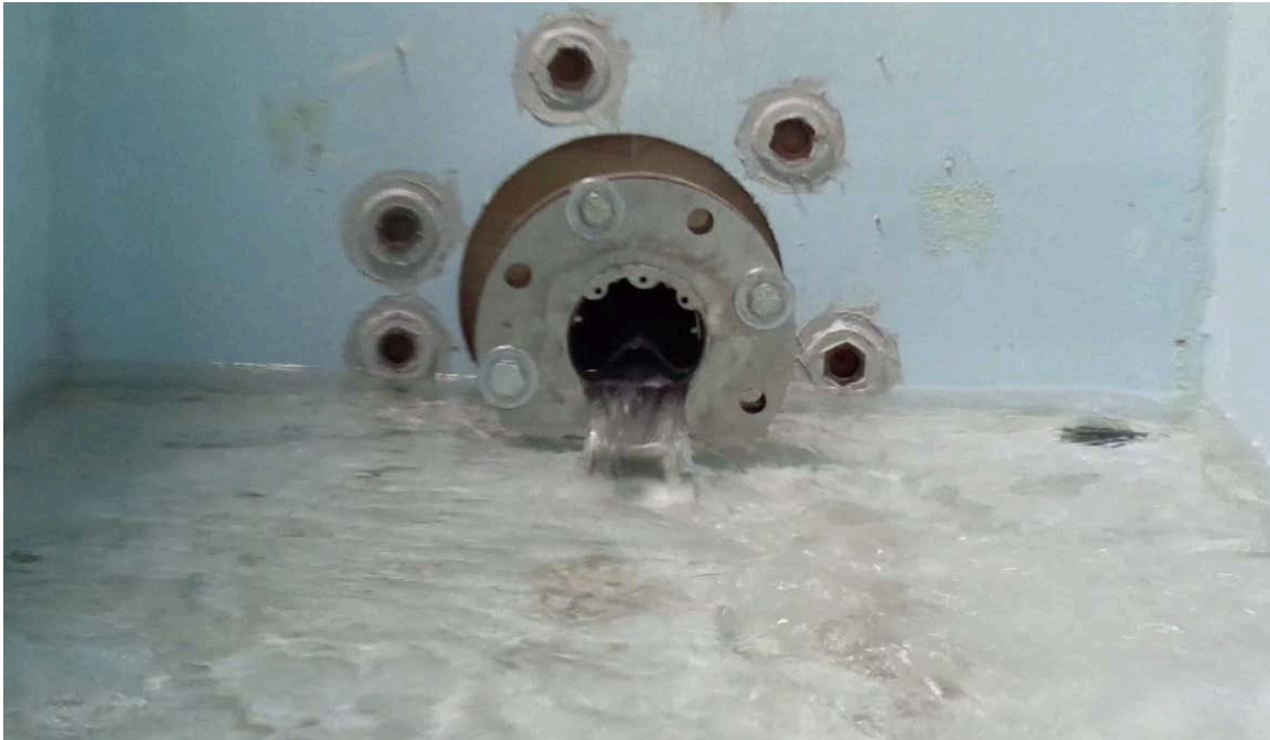
Figure 1. Test Setup for the Free-Discharge 4-Inch Rubber Check Valve Tests
